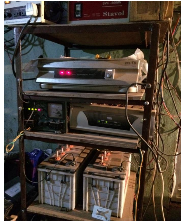
Fig. 11: Power Backup System of MICET before EQ
